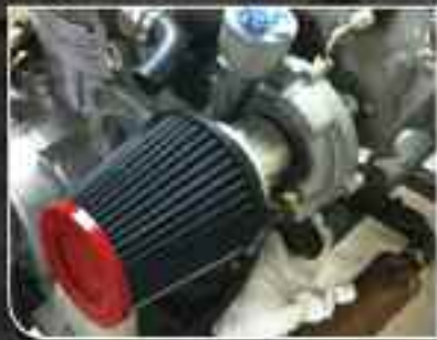
FLAME ARRESTOR #S9-2040RR INSTALLED
